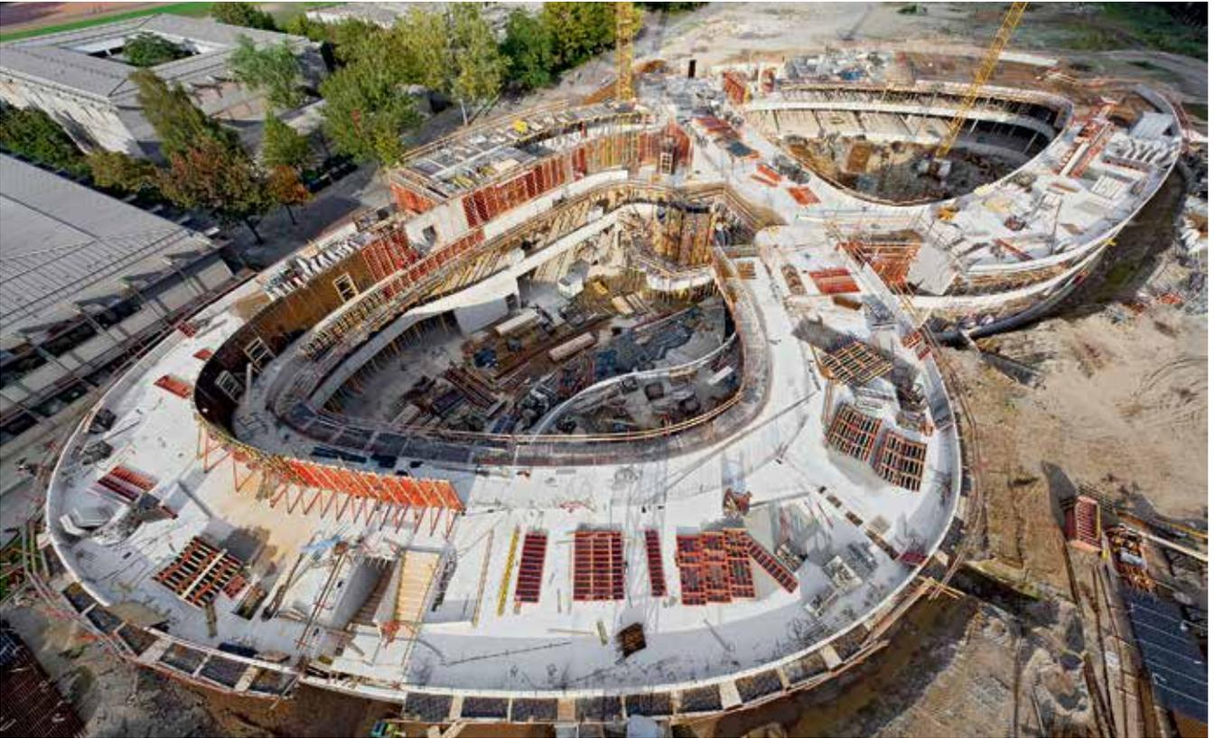
**RUNDFLEX is an enormously versatile and adaptable circular wall formwork. The system provides a solution for virtually any challenge in connection with curvatures, changing radii, roundings and arches.**
