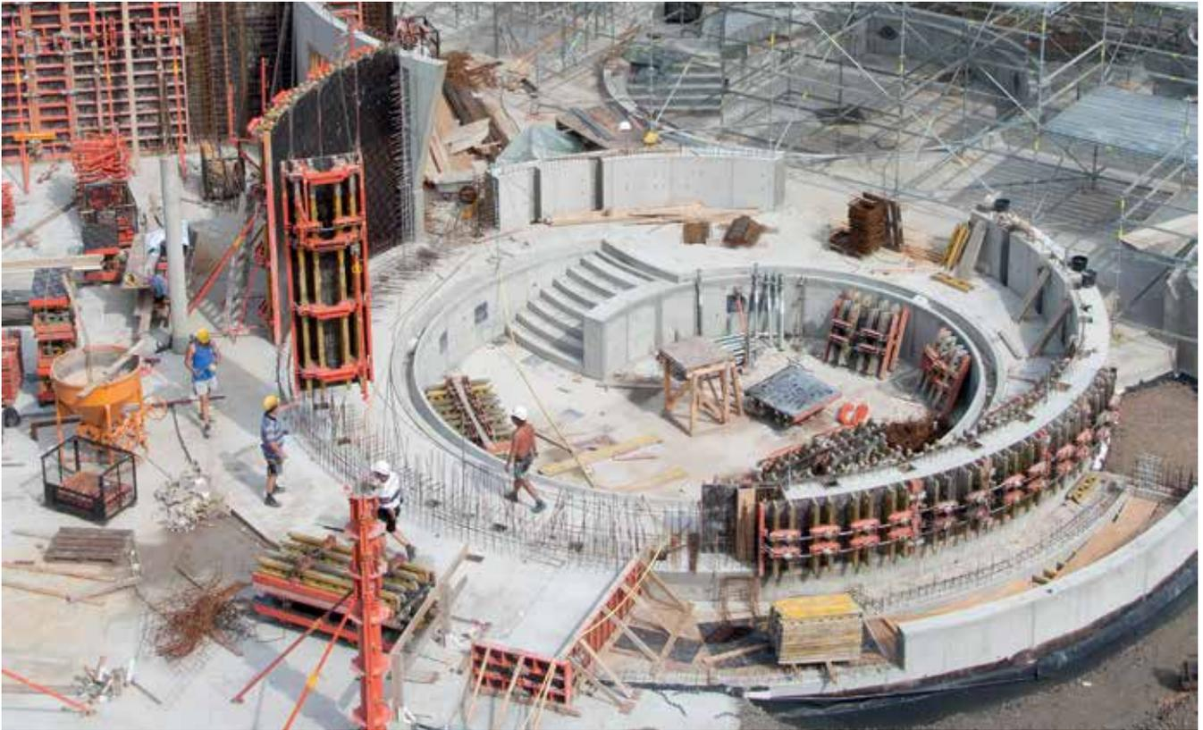
**RUNDFLEX elements are pre-assembled at the assembly hall and are available in 3 different panel widths and 6 panel heights.**
