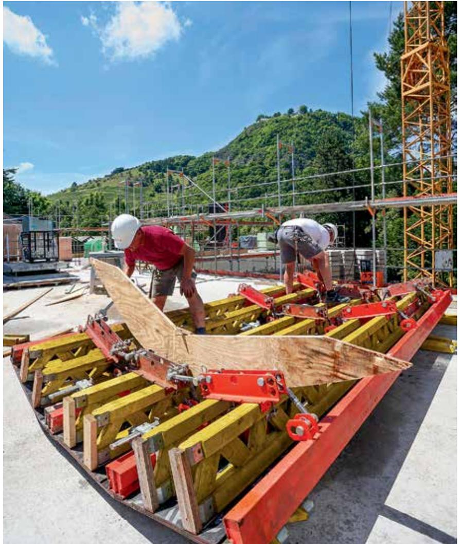
Checking the required curvatures is carried out by placing the radius template on the formwork girders.
