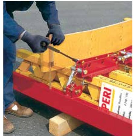
The adjustable spindle for adjusting the edge profile is also operated by means of the "combi" Ratchet Spanner.
