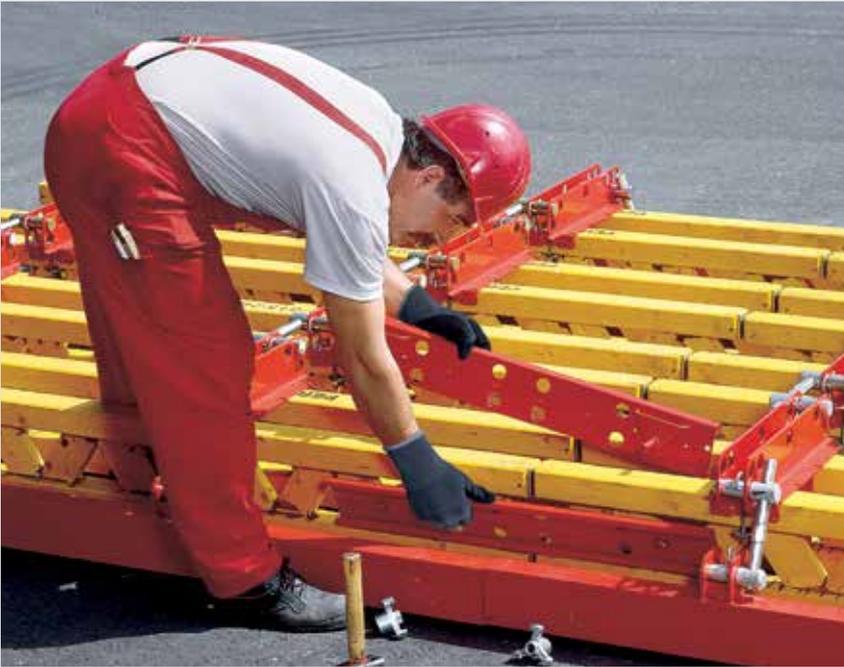
**RUNDFLEX elements can be extended in 60 cm increments.**
